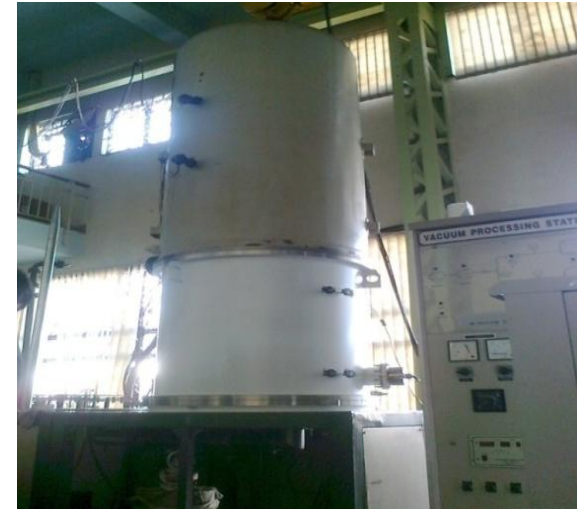
Vacuum Processing Unit
